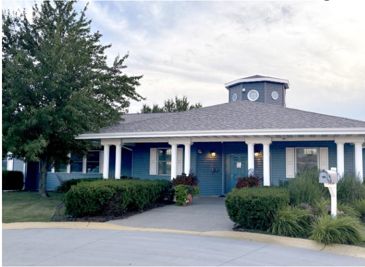
St. Jude House Domestic Violence Shelter and Prevention Center in Crown Point, Indiana.
